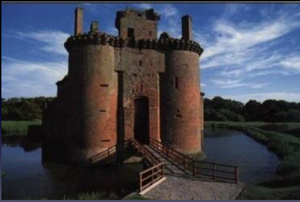
Breaching the Gate
